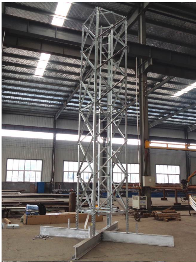
117a). View of the tower ready for the shield installation.
