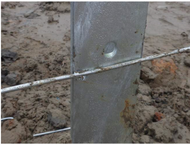
26). The tension wire must pass from outside of the intermediate posts as indicated here
