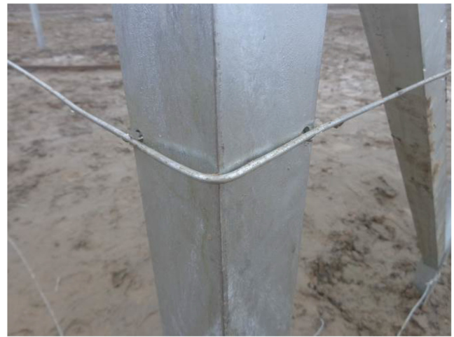
27). The tension wire must pass from outside of the corner post as indicated here
