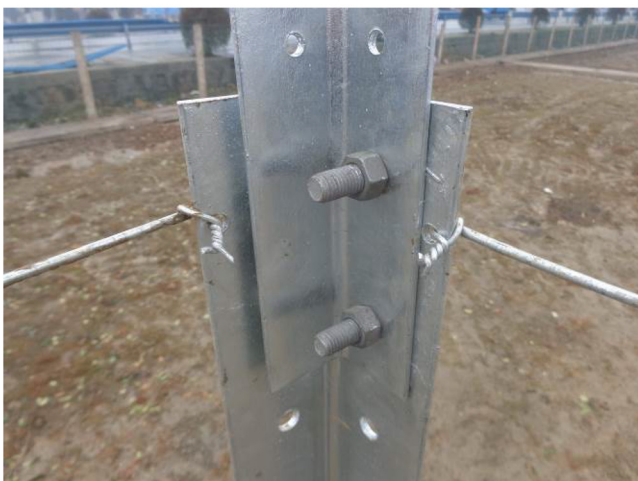
76). Inside view of corner post &amp; razor wire support
