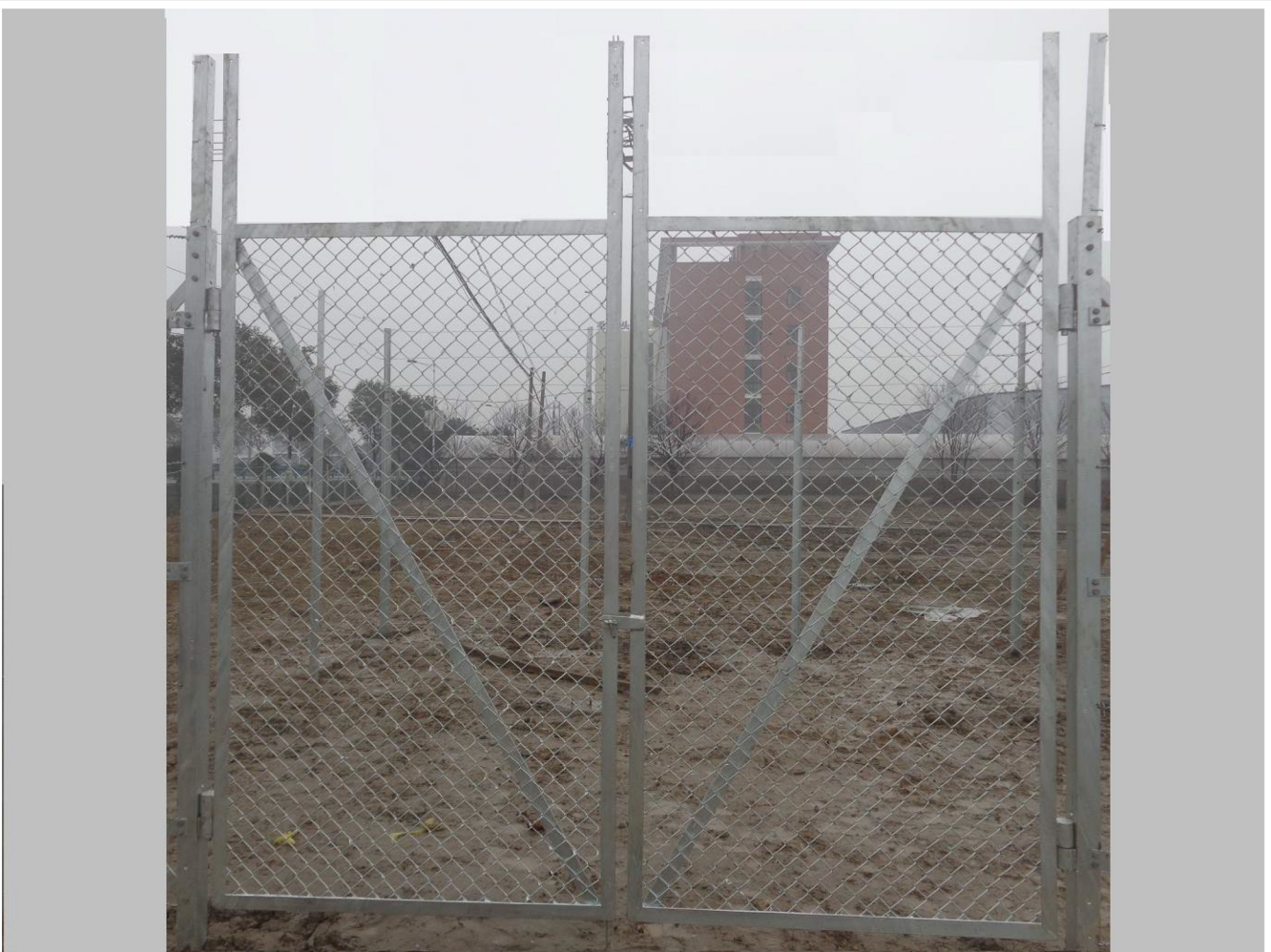
22). Gate is installed and secured
