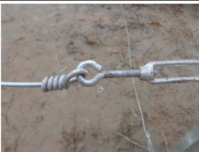
24). Connect the tension wire to the tensioners as described here or in a similar way
