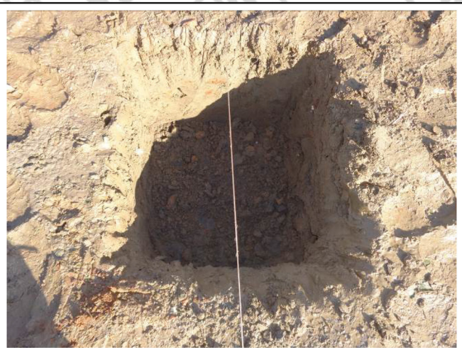
06). Use the plumb bob again to verify the depth of each excavated hole
