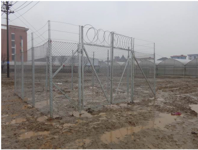
74). 6 x 6 site view, partially complete
