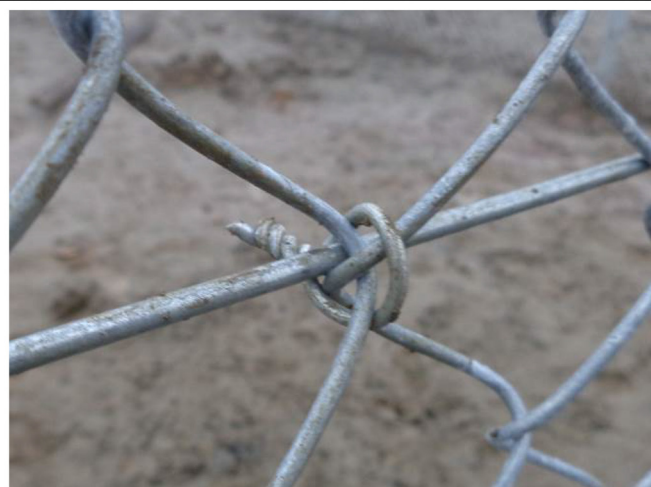
50). View from Outside the fence. A typical way of connecting the chain-link mesh to the tension wire
