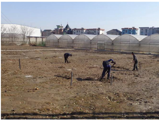
01). After nominal ground zero decided upon, starts by setting up the spikes and string.
