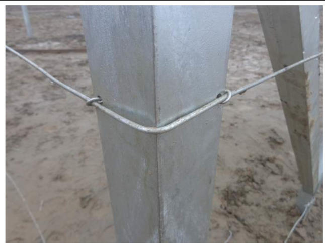
37). Tighten the small pieces of wire after all tensioners are tightened (View from outside)
