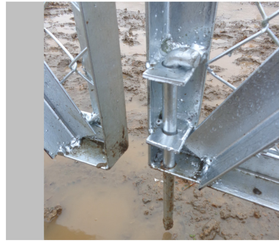
21). The gate is supplied with a drop bolts indicated here
