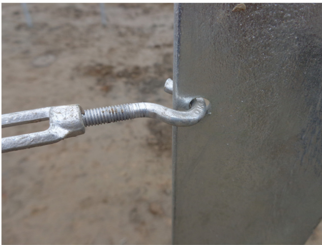
28). Connect the tensioners to the posts and razor wire support as described here or in (Pic.29)
