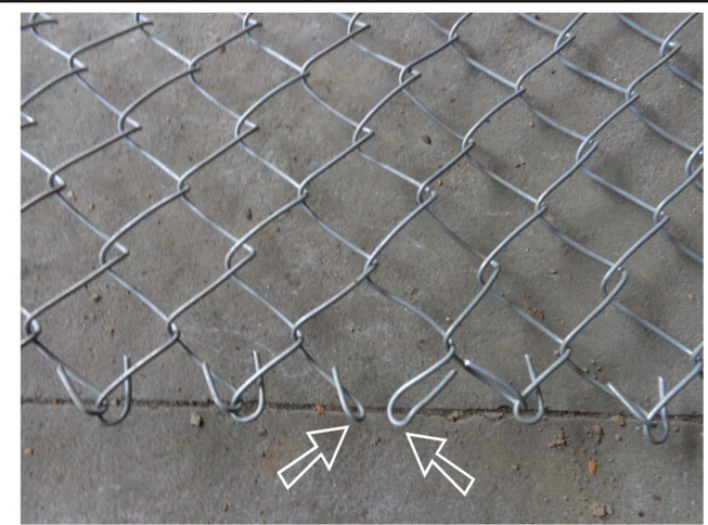
56). After you have successfully woven the two rolls together, re-knuckle the ends together
