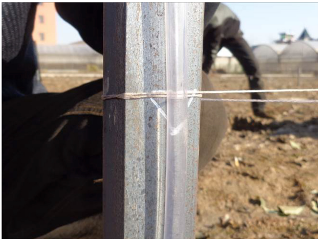
03). Make sure the string is levelled and mark each post location with a plumb bob
