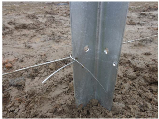
33). PRIOR tensioning the wire, put small piece of wire as indicated here but DON'T tighten them.
