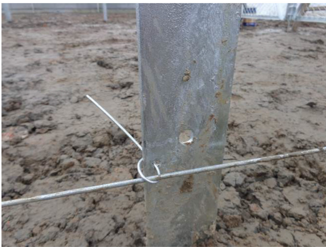
32). PRIOR tensioning the wire, put small piece of wire as indicated here but DON'T tighten them.
