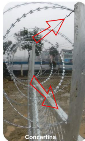
79). View of installed razor wire.
