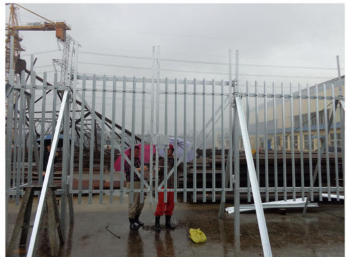
Trial of Palisade fence – 3m Gate
