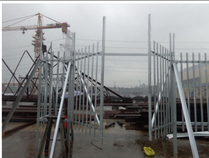
Trial of Palisade fence
