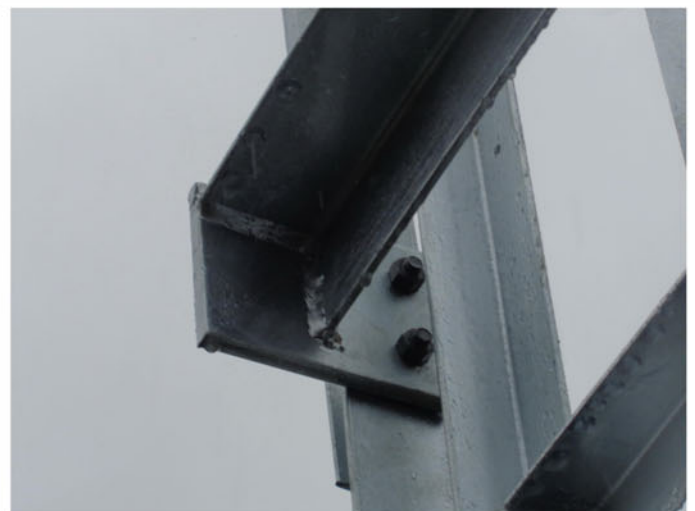
Trial of Palisade fence – Top gate beam
