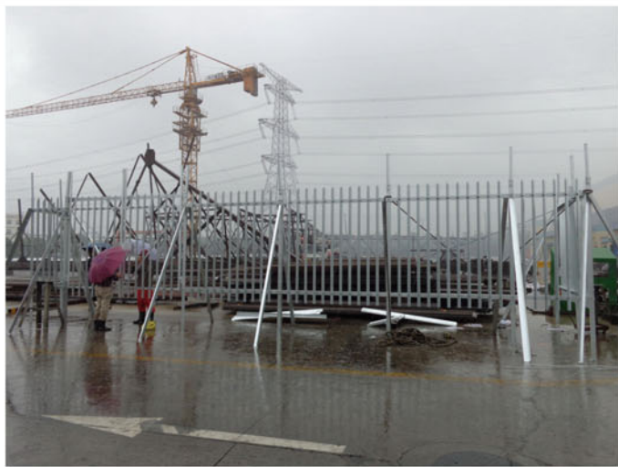
Trial of Palisade fence
